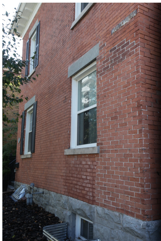
Northeast corner of 524 Clarence, showing possible indication that the window was formerly a door
