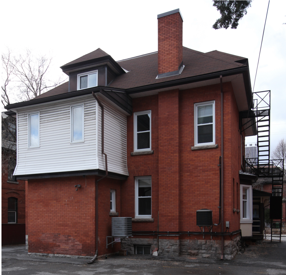
Backstairs. The vinyl siding upstairs suggests that this may originally have been a sun porch. In the renovation of 1963 it was enclosed and converted into a “lounge”.
